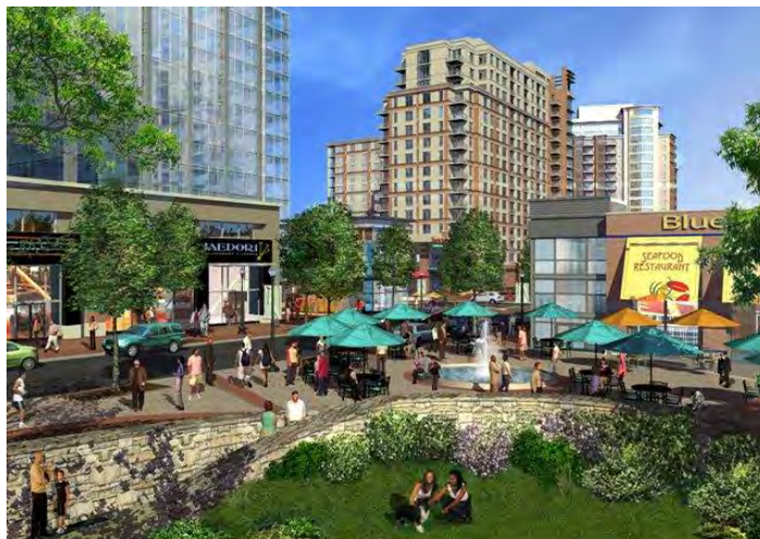
North Bethesda Center is one of five flagship projects clustered along Rockville Pike in White Flint.
