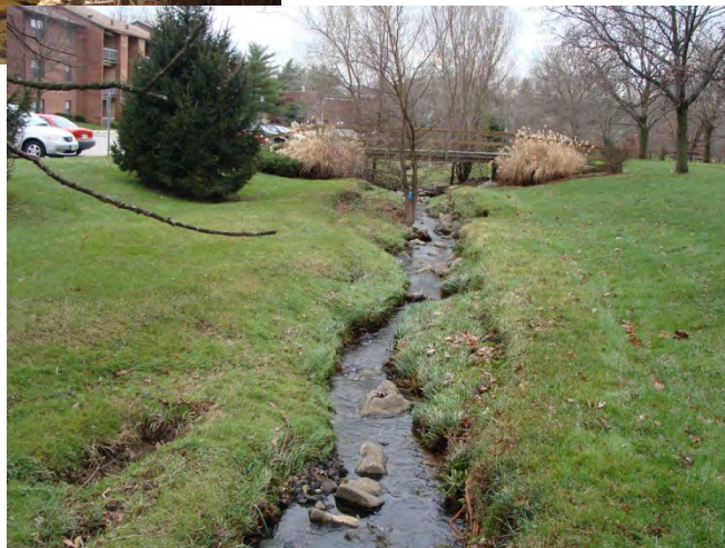
Beaver Dam after - Plantings secure the banks to prevent sediment and nutrient pollution. The roots absorb the nutrients to help the plant grow and the roots hold the soil in place.
