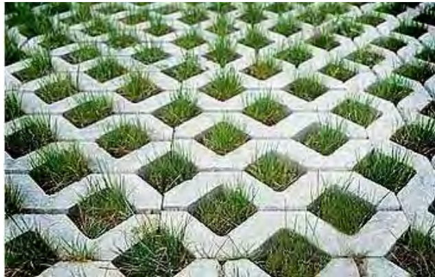
Permeable pavers allow water from rain to flow through traditionally impervious paved surfaces into the ground thereby reducing run-off to streams
