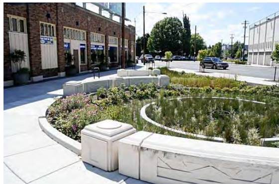
Innovative street features, such as that pictured, provide aesthetically pleasing streets as well as help to take stormwater off the streets and into the ground
