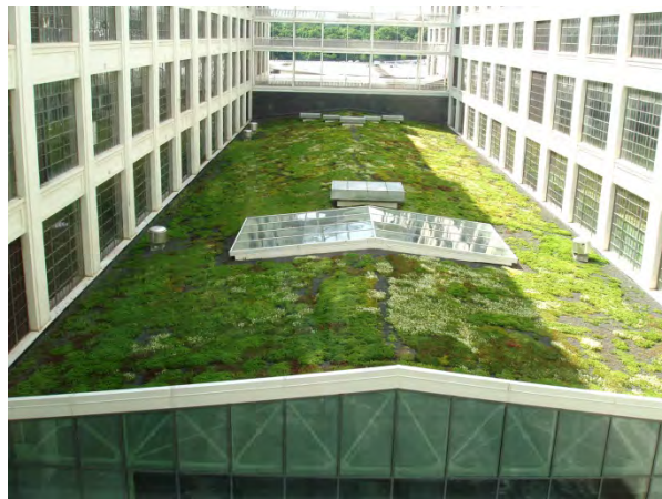
A green roof is partially or completely covered with vegetation for the purpose of absorbing rainwater, providing insulation, creating a habitat for wildlife and helping to lower urban air temperatures and mitigate the heat island effect.
