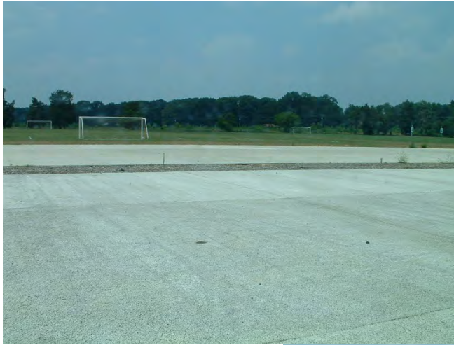
Bloomfield Parking before - Asphalt or concrete heats run off and quickly transports it to local streams. Excessive heat and velocity are bad for local waters.
