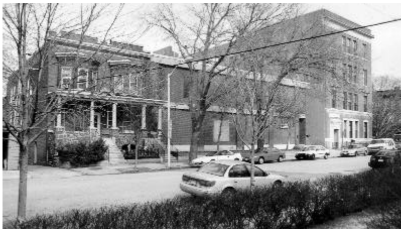
CONTEXTUAL CONSIDERATION. THE MIDDLE BUILDING WAS BUILT IN 1926, 13 YEARS AFTER THE ROWHOUSES. THE CORNICE BAND AND PORCH LINE IS CARRIED ACROSS THE NEW FACADE, RESPECTING THE PRESENCE OF THE HOUSES, BUT THE LACK OF FENESTRATION PRESENTS A BLANK FACE TO THE STREET
