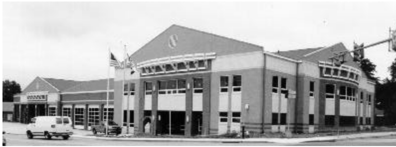
THE NEW FIRE STATION ON THE EDGE OF DOWNTOWN BEL AIR, MD IS PULLED UP TO THE BUILDING LINE
