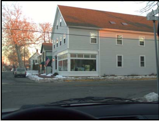
Adaptive reuse suits in-town commercial development
