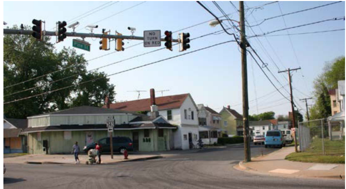
The intersection of Pine Street and Washington Street (MD Route 343) lacks serious attention to the safety of pedestrians. .
