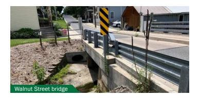
In 2013, the bridge on Walnut Street over Tanners Run was replaced due to its deterioration over time. The bridge is located approximately 500 feet from the intersection of Walnut Street and West Main Street. In addition to the replacement of the superstructure and the rehabilitation of the bridge abutments, roadway approaches and storm drainage improvements were made as well. See Map 5-1 following this chapter, Roads by Jurisdiction map.
